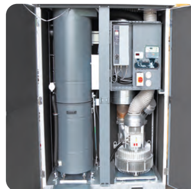
Inner workings of the CENTRAL CAR CLEANING SYSTEM
